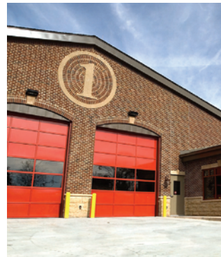
New Fire Station 1
