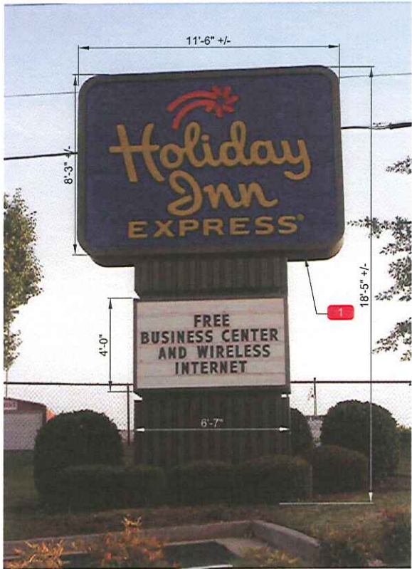
Existing Double-Faced Internally Illuminated HI-12 Pylon Sign (95 sq. ft.)
