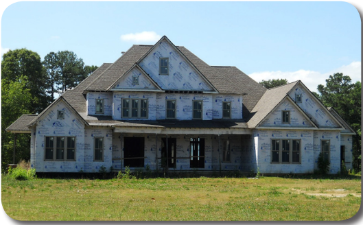
Poorly maintained vacant structure
