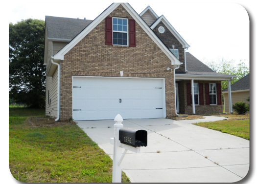
Properly maintained vacant structure
