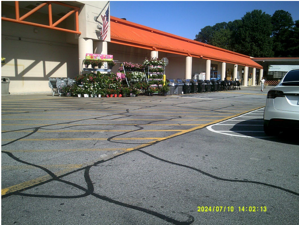
View of front display area
