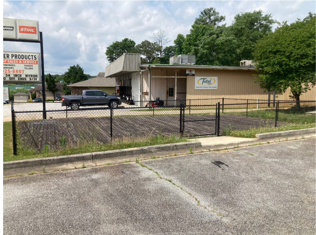
View of existing detention pond
