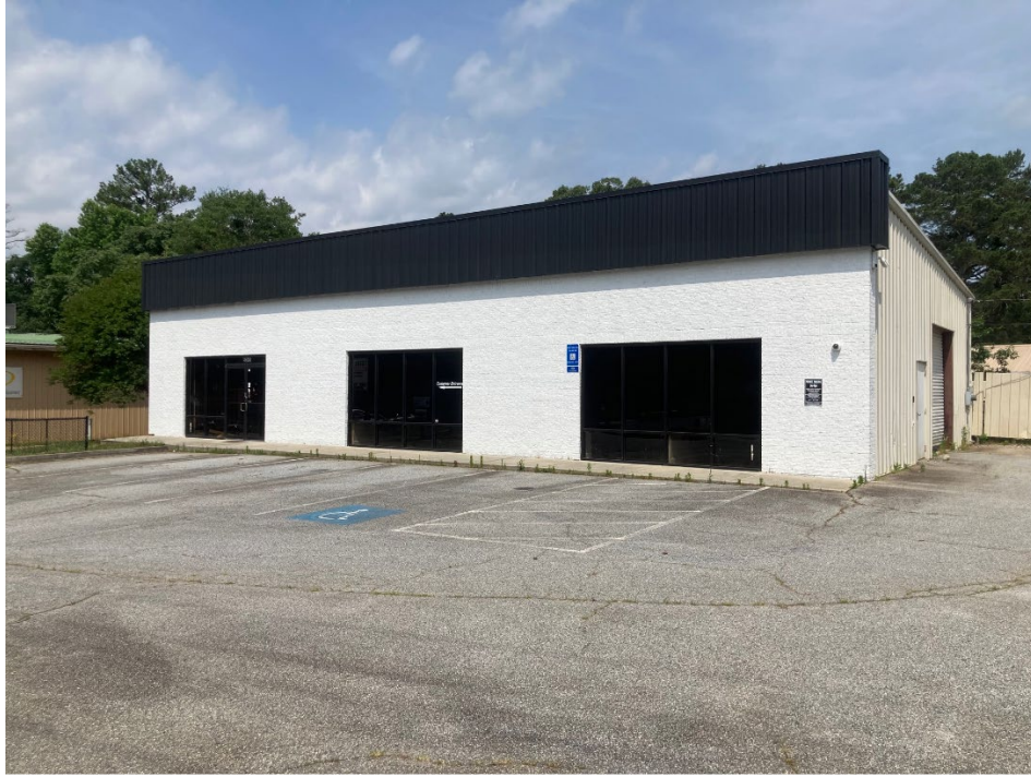
View of existing building on the subject property
