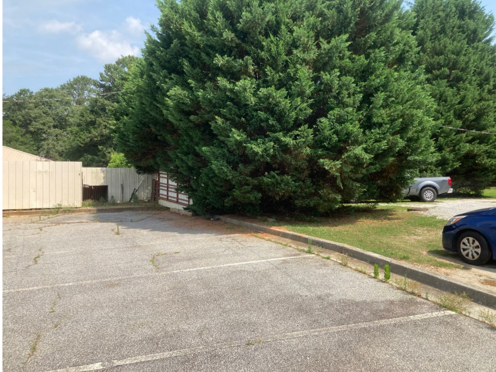
View of existing parking available and potential location for interparcel access
