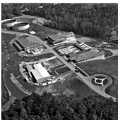
Shoal Creek Filter Plant
