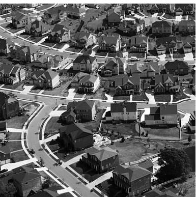
New Home Construction
