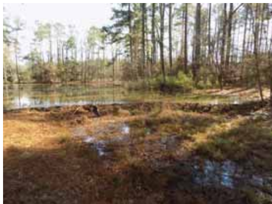
Emergency spillway (active flow / seepage)
