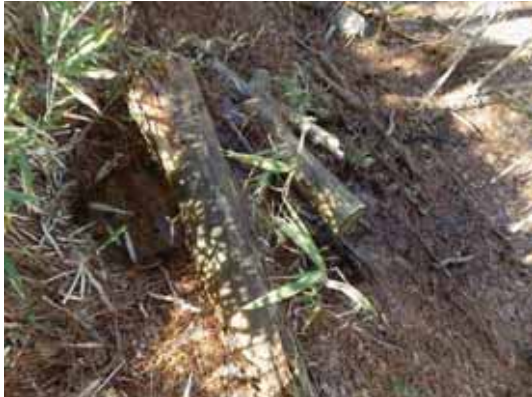
Hole with active flow through dam
