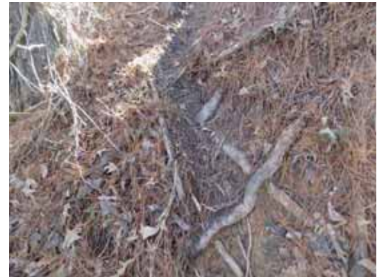
Signs of erosion on downstream slope from overtopping
