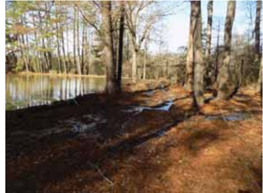
Northeastern corner: overtopping / seepage
