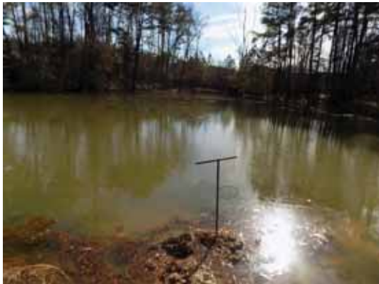
Clogged outlet structure / valve
