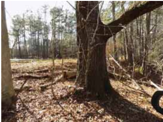
Mature tree on downstream slope of dam
