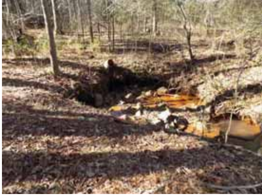
Stagnant plunge pool from clogged / damaged outlet
