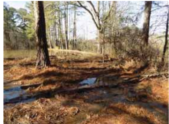
Northeastern corner: overtopping / seepage
