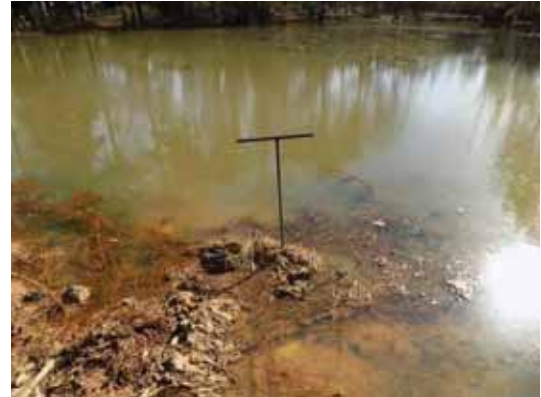
Clogged outlet structure / valve
