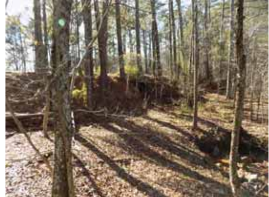
Mature trees on downstream slope of dam
