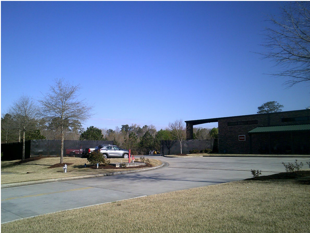
View from Athens Highway of Fenced Storage Area
