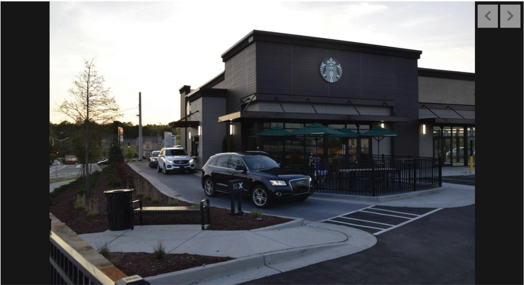
Customers go through the drive thru at the new Starbucks located in The Exchange at Gwinnett mixed-use development on Buford Drive at Interstate 85 on Monday.
