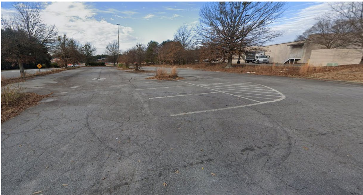
View of the rear parking lot
