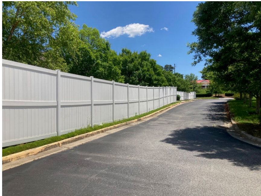
View of the interior driveway and privacy fence
