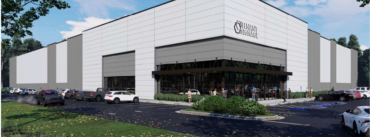
Below is rendering and material is PEMB structure with a mix of horizontal and vertical IMP (Insulated Metal Panel) skin. There are many colors available.
