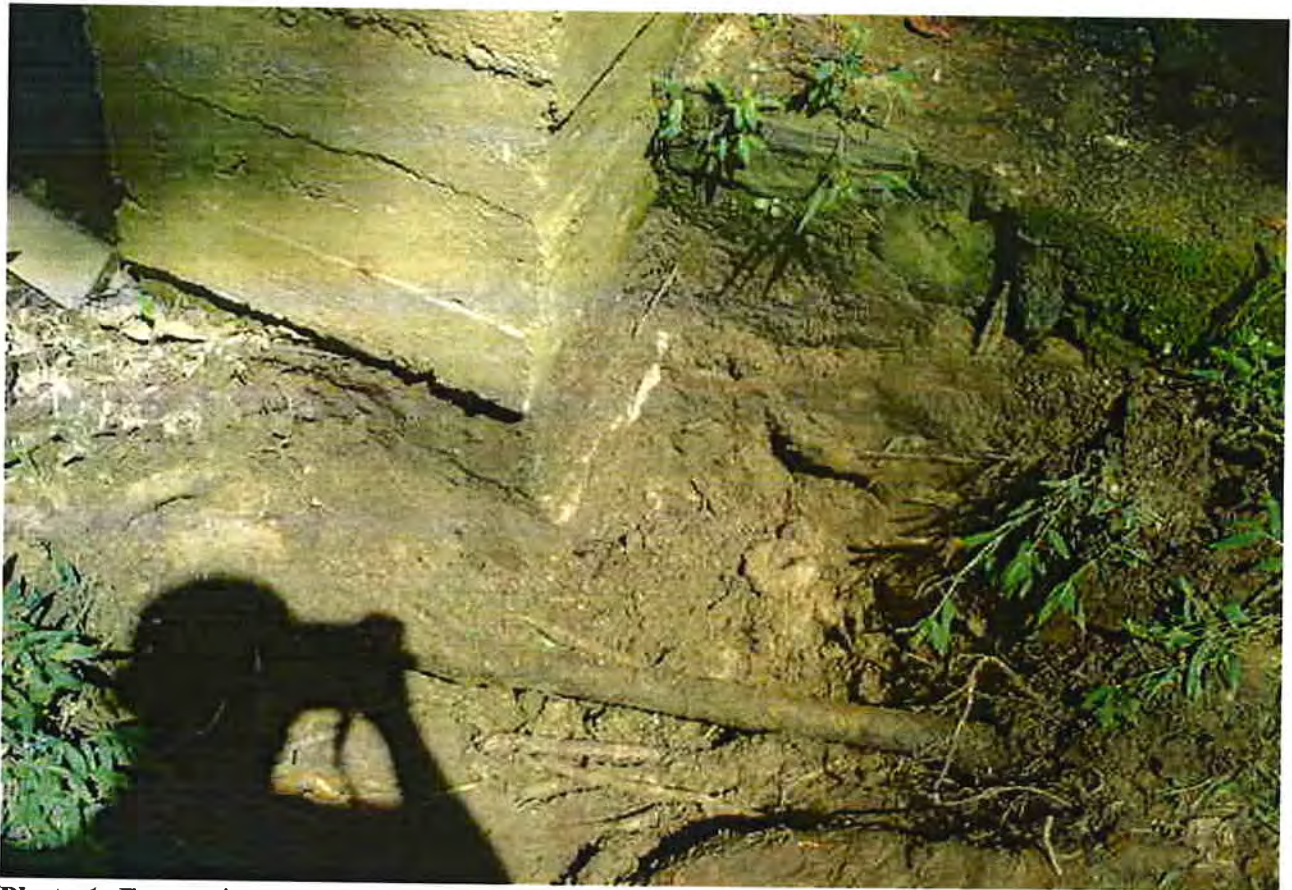
Photo 1: Excavation at column #2
