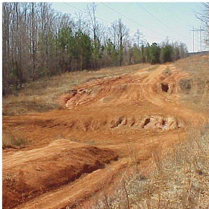
*Widespread Erosion Ruts at Georgia Power Easement*
