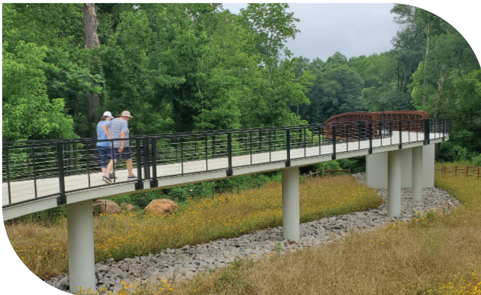
Figure 52. Elevated concrete boardwalk with pedestrian bridge for grade-separated crossings- North Oconee River Greenway-Athens, GA.
