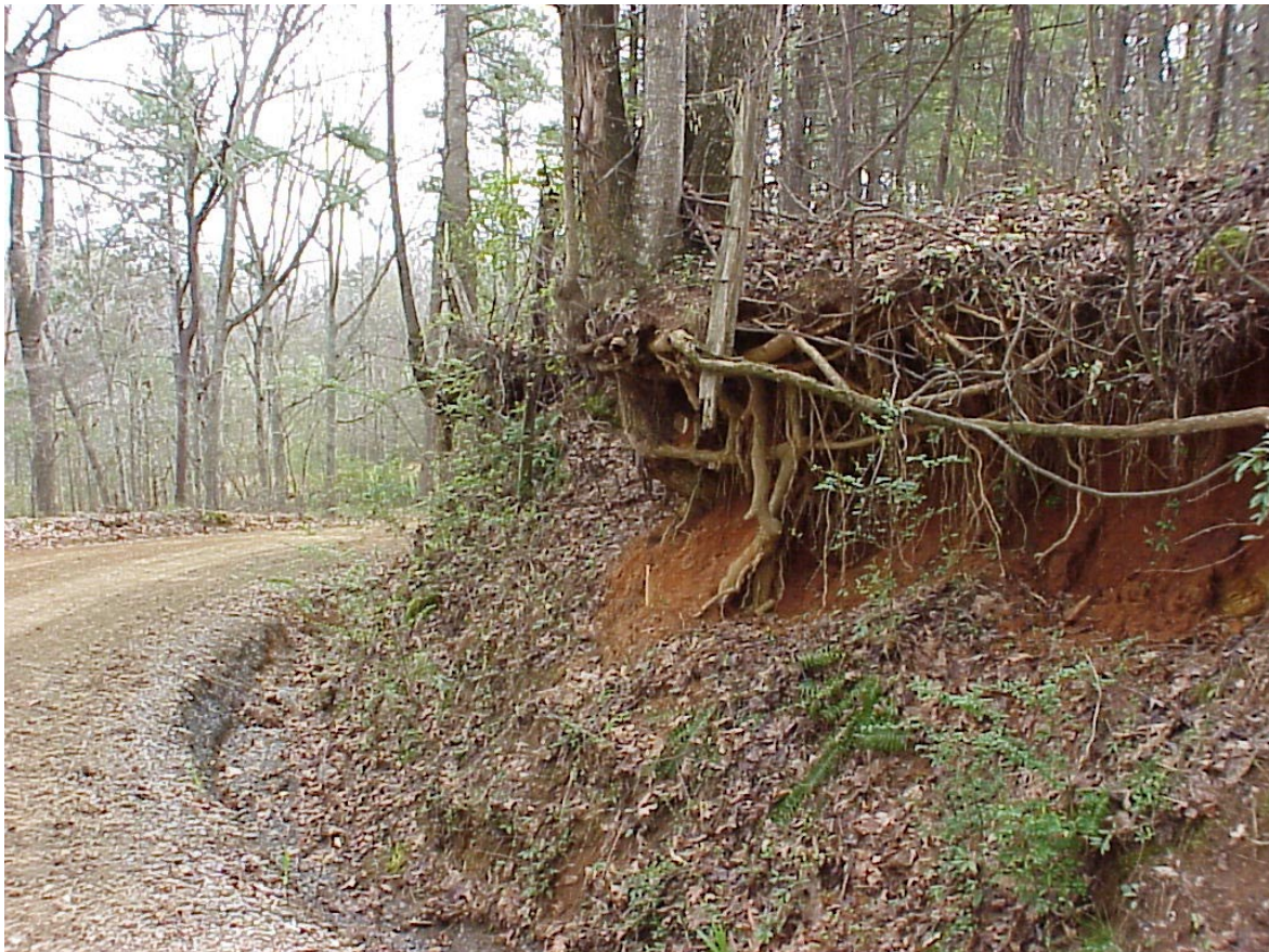
Severely Eroded Embankment at McDaniel Farm Road – Section to be Re-aligned
