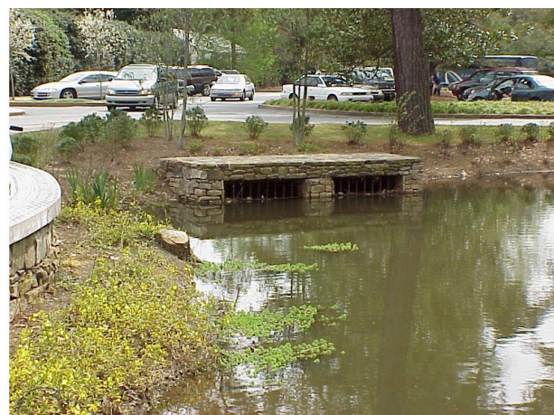
Appropriate Marginal Planting and Outlet Control Structure Detailing, Sibley Hortic. Center, Calloway Gardens
