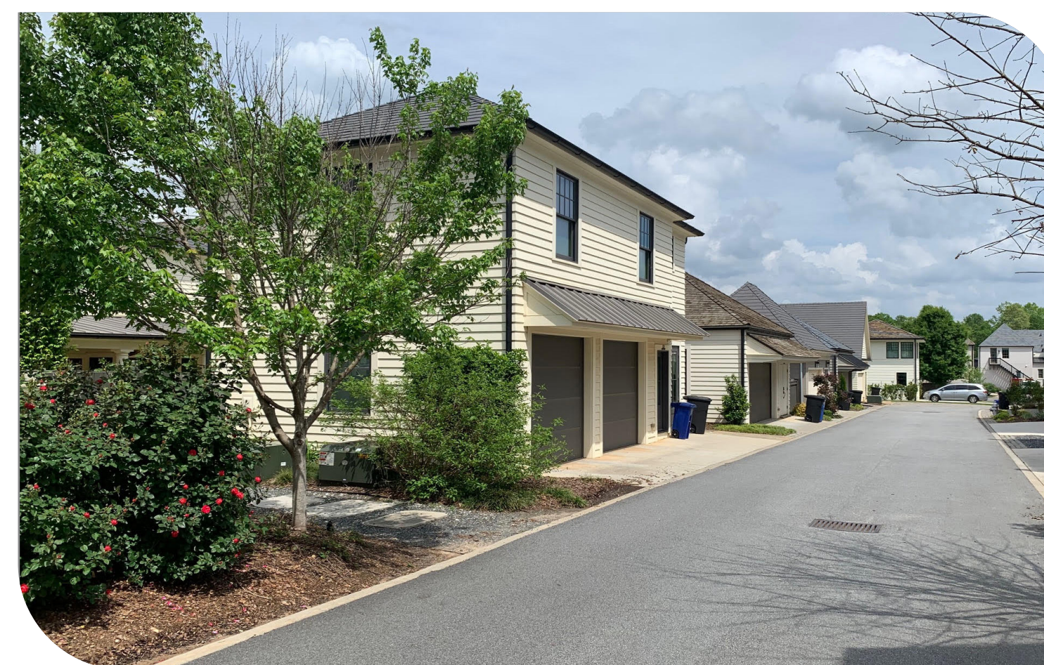
Alley access to parking
