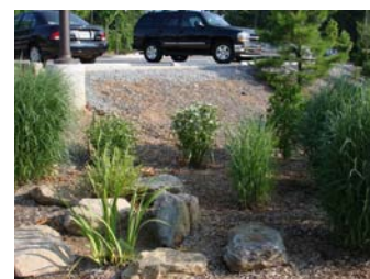
Figure 10: Bioswale
