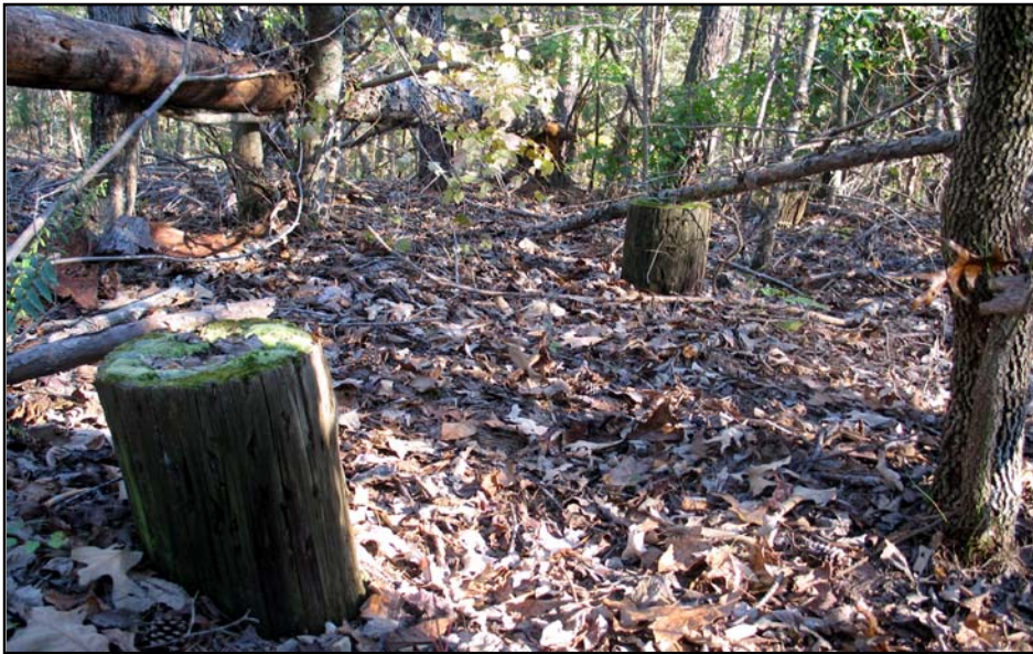
Figure 11: The wooden piers shown here were formerly used to hold a small farmhouse up off the ground.
