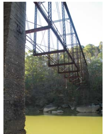
View of Settles Bridge without Decking
