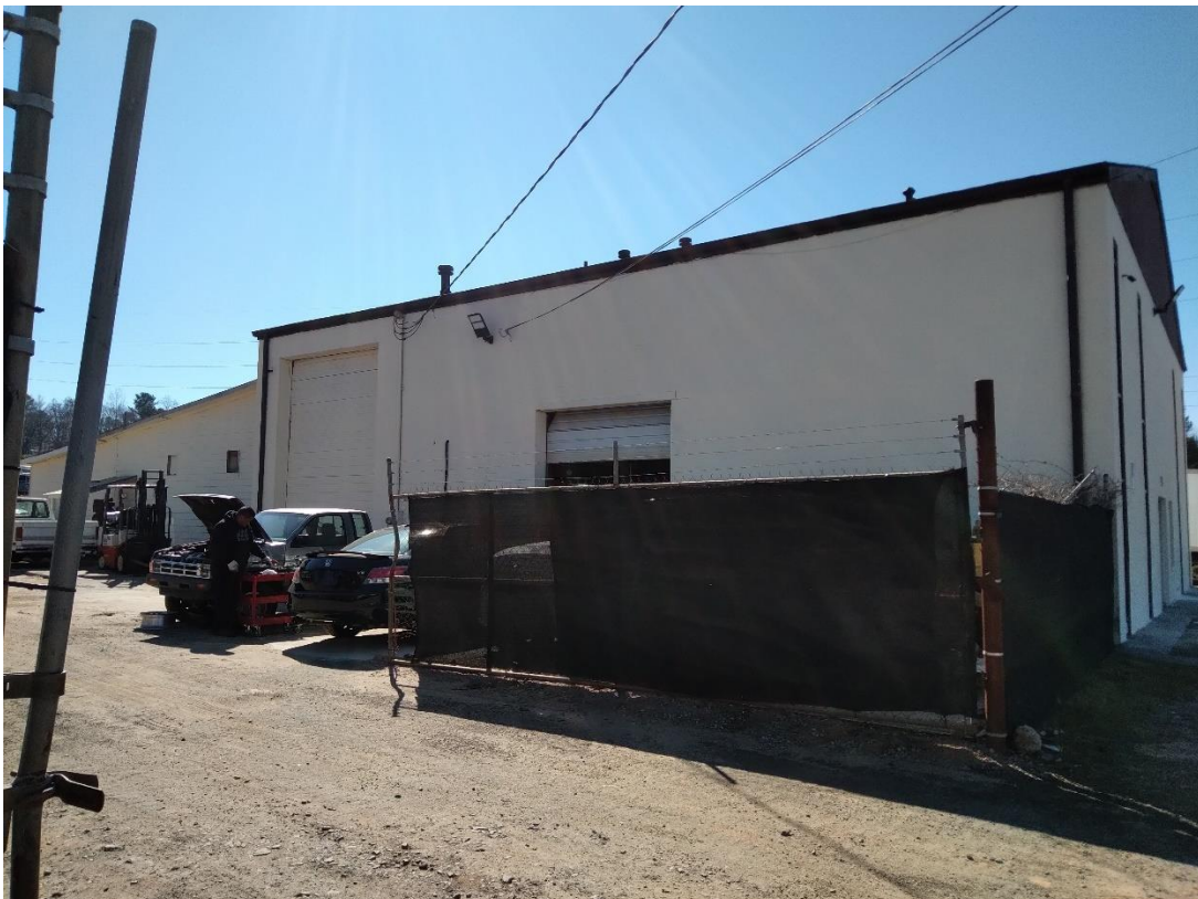
Bays on east side of building
