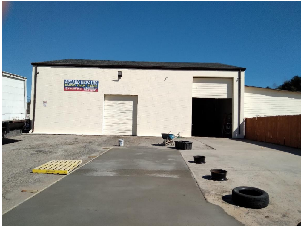
Bays on west side of building along Arcado Road
