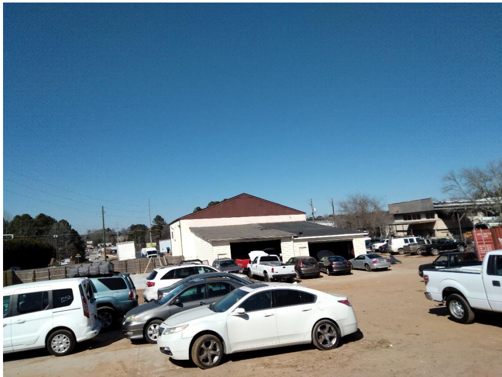
Rear of building
