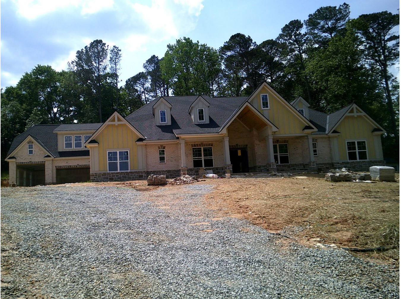
Single-Family Residence Under Construction
