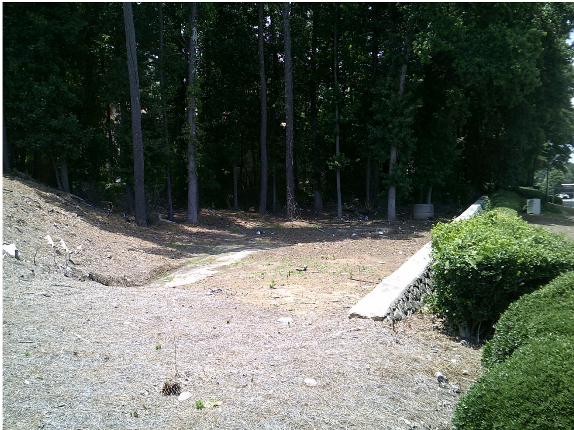
Existing stormwater management facility along right of way
