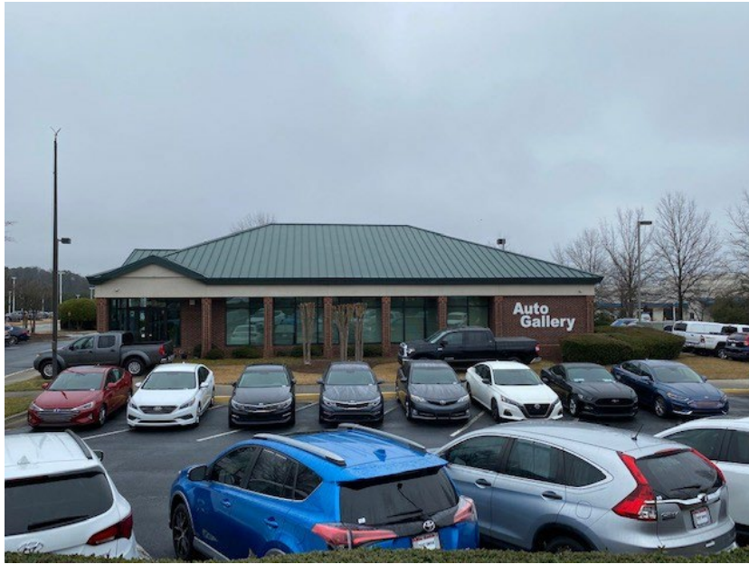
SITE VIEW FROM SATELLITE BOULEVARD
