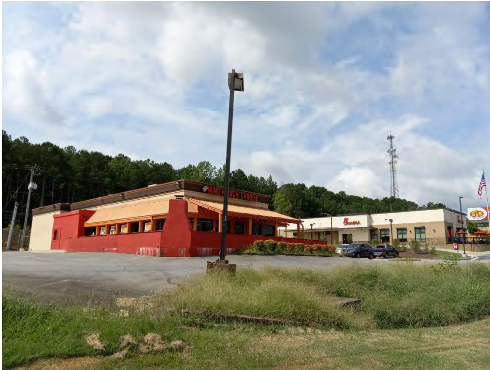
Existing restaurant building
