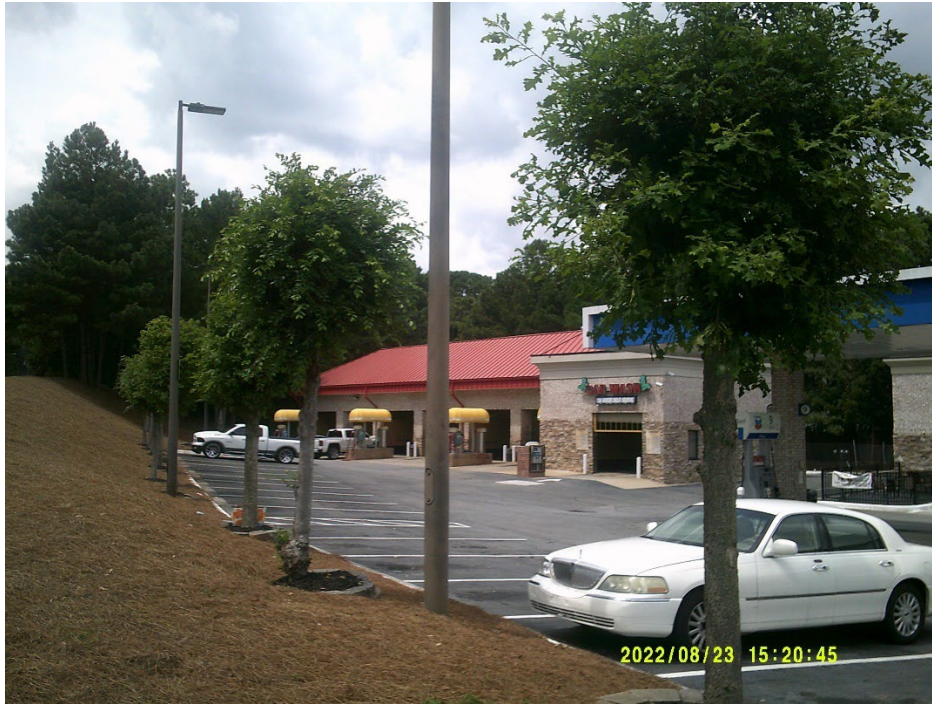
Existing self-service car wash
