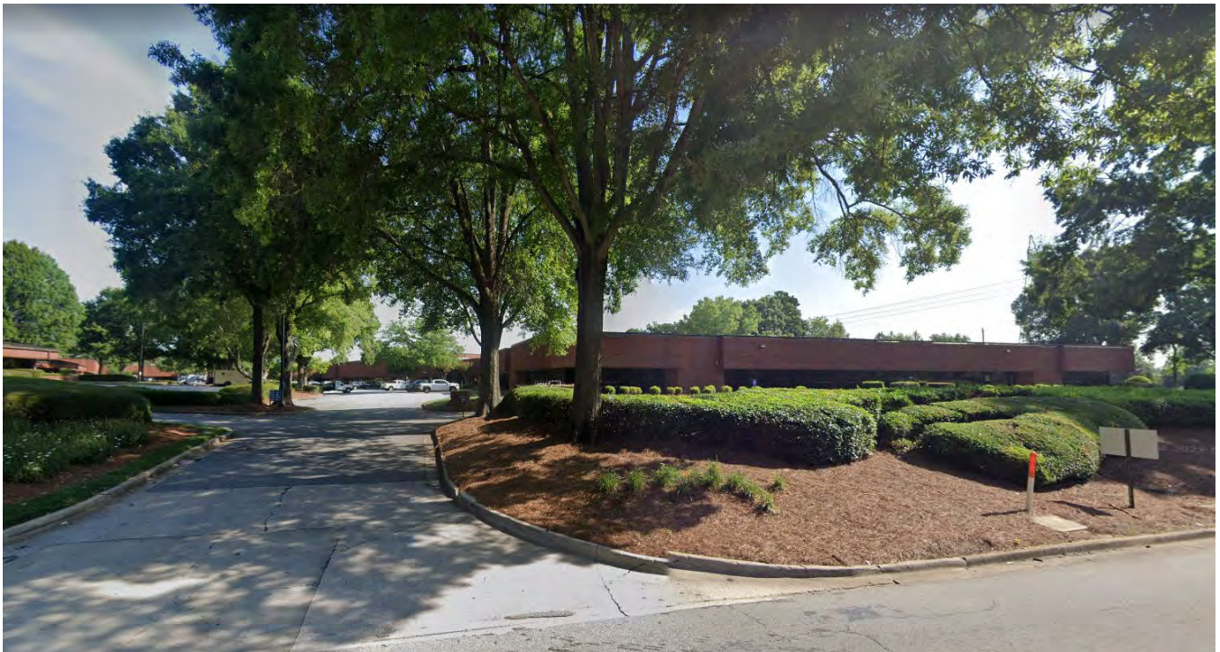
Existing Driveway to Serve Proposed Adult Day Care Facility
