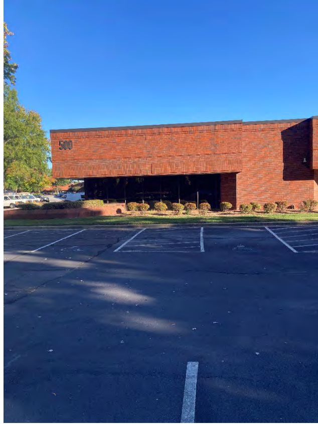
Front of Building 500
