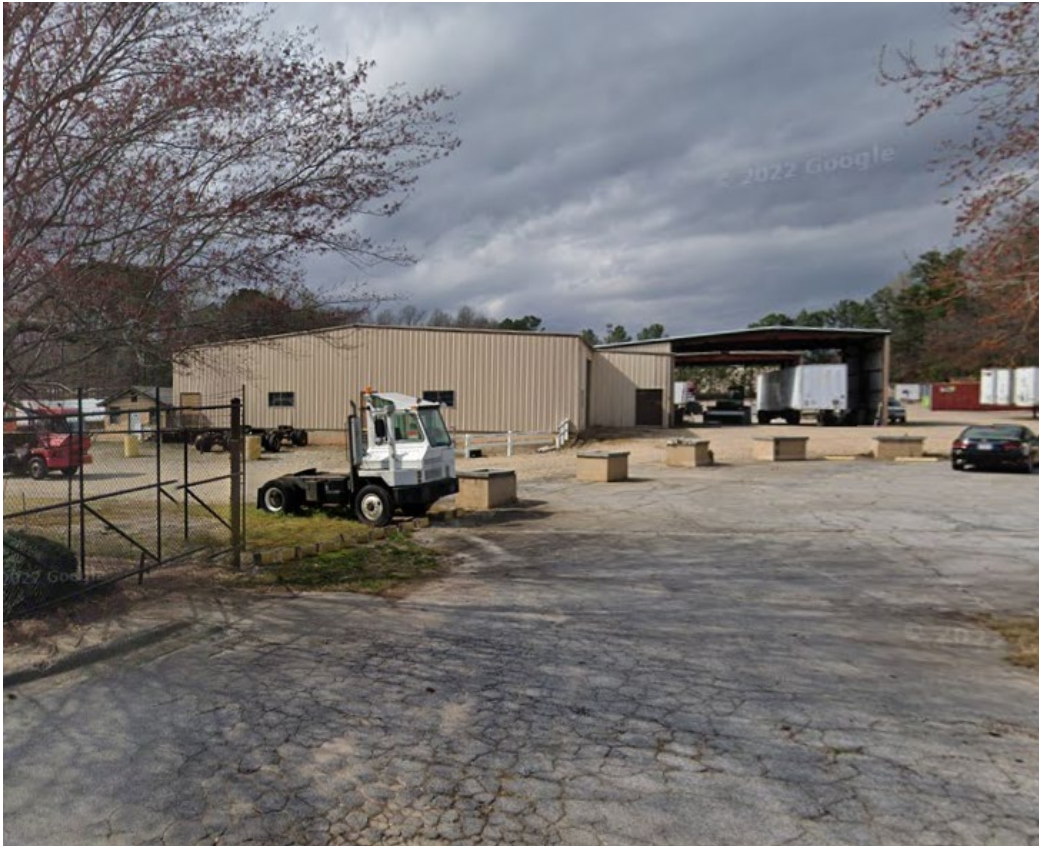
View of metal building and gravel parking area from Hurricane Shoals Road
