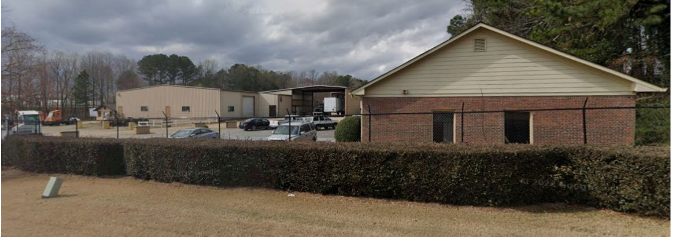
View of the office building and metal building from Hurricane Shoals Road
