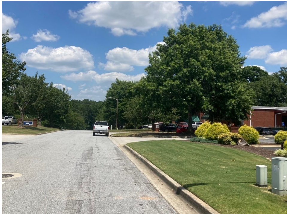
View of site access and Hewatt Court road frontage
