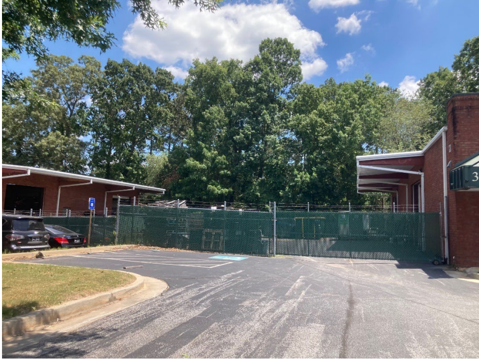
View of the enclosed parking area
