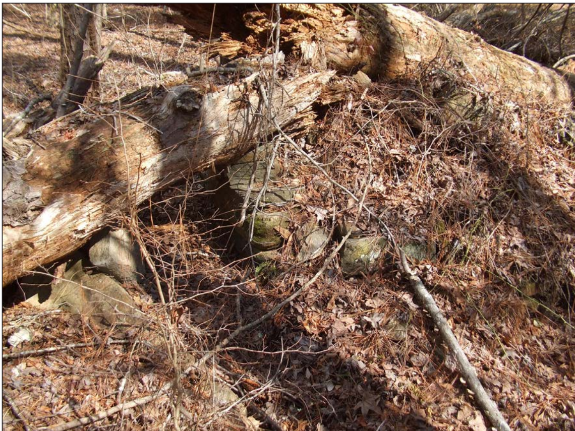
Figure 11. General view of TPG-3, northwest chimney fall, facing east
