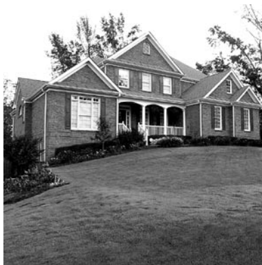
New Home Construction
