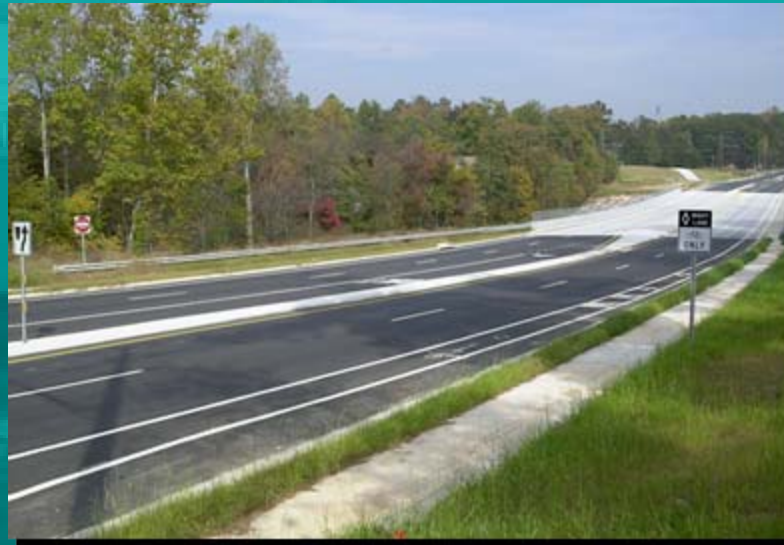
Annistown Road widening
