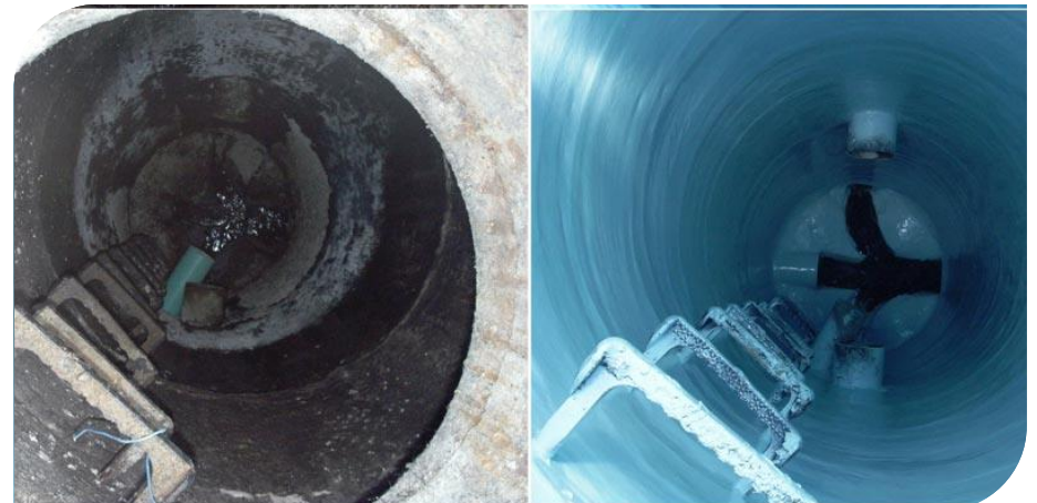
Manhole/Structure repair and rehab
