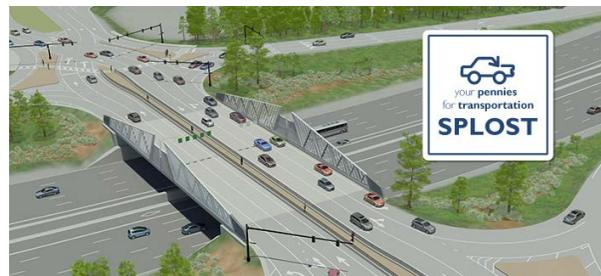
The design uses the existing bridge more efficiently by switching traffic to the left to allow smooth
