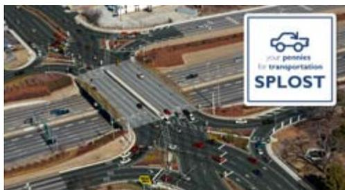
The DDI's innovative design relieves congestion, improves safety, and is less expensive than replacing or widening the bridge. A DDI shifts traffic to the opposite side of the road, making left turns onto the interstate easier and improving the flow of traffic across the bridge. Find out more about the projects at [www.gwinnettddi.com](http://www.gwinnettddi.com).
