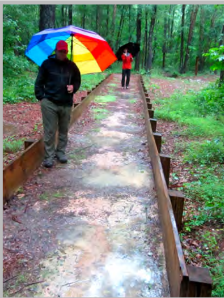
Right: Fall line trail with multiple flow rills, no attempt at water management
