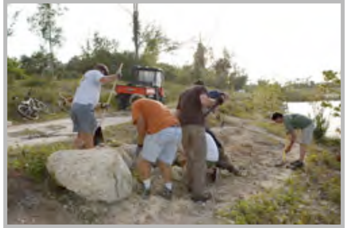
Balance features, constructed of wood or rock, with managed fall zones adjacent to a trail
