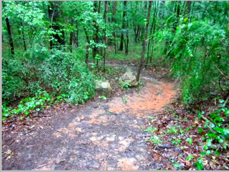
Left: Fall line trail, eroding over a width of 6' and depth of 9"
