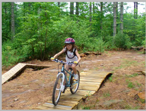
Balance features, constructed of wood or rock, with managed fall zones adjacent to a trail
