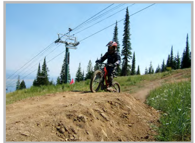
Challenge features, that allow riders with the skills to jump/drop, constructed within the trail tread and at the same difficulty level as the remainder of the trail
