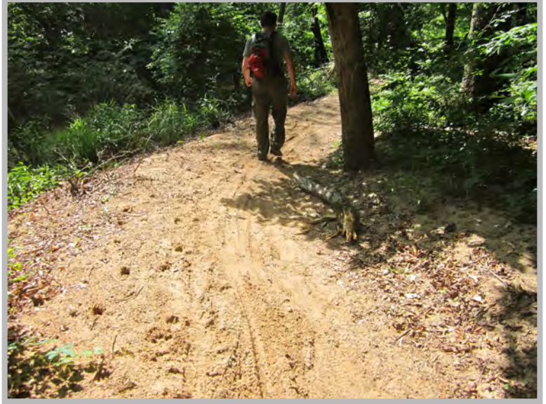
Left: Fall line alignment makes maintenance very difficult
