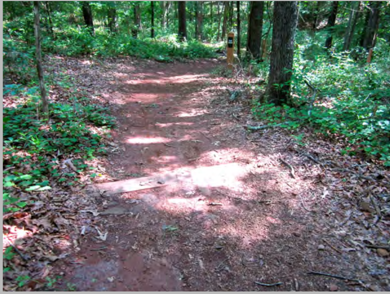
Left: Large water bar, completely filled by sediment
