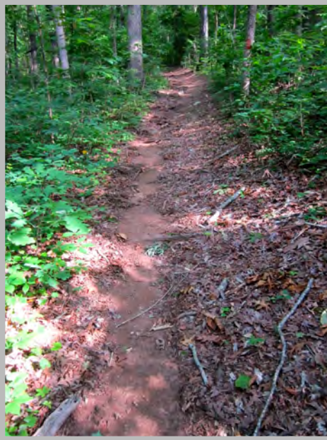
Left: Fall line trail with indications of incision- organic debris removed from path of flow
