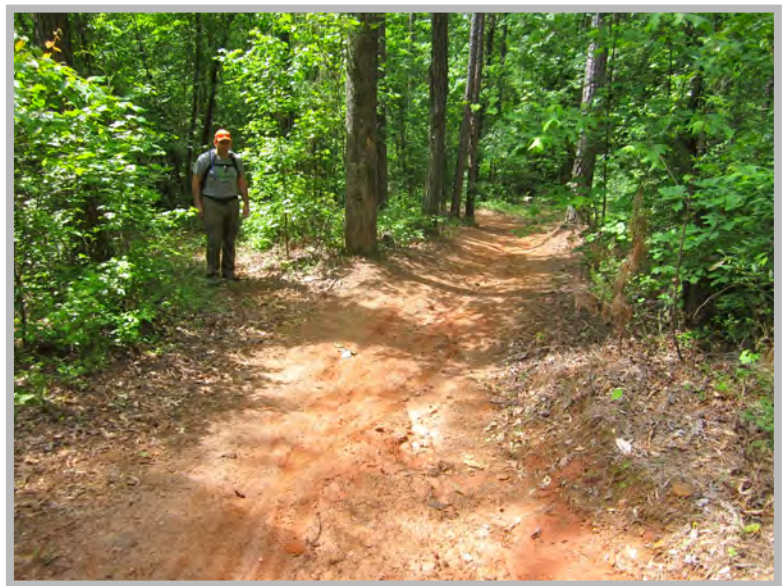
Left: "Turnpike" structure, ~9" unfilled and without drainage
