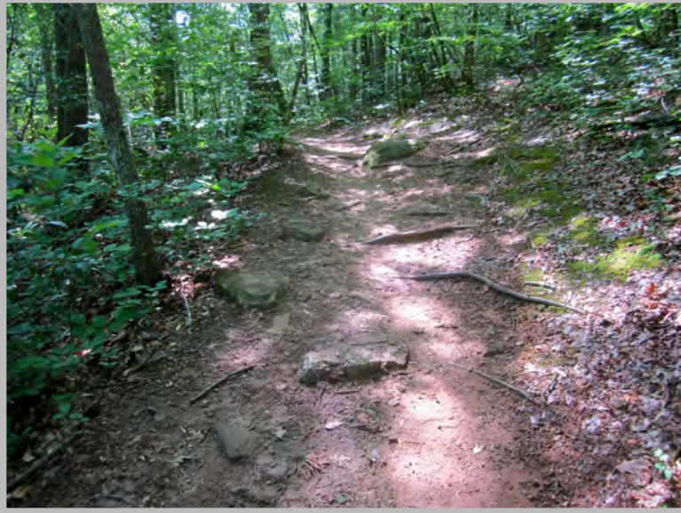
Left: Fall line trail, widening as obstacles become larger as soils are further eroded
