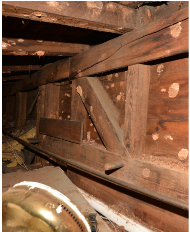
Figure 6: Mortise and tenoned timber framing.
