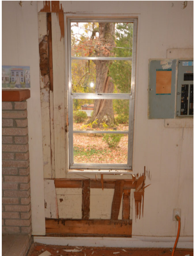
Figure 12: Aluminum window in a larger opening. Note the corner bead wood trim, removed sill/stool, and wainscot below.
