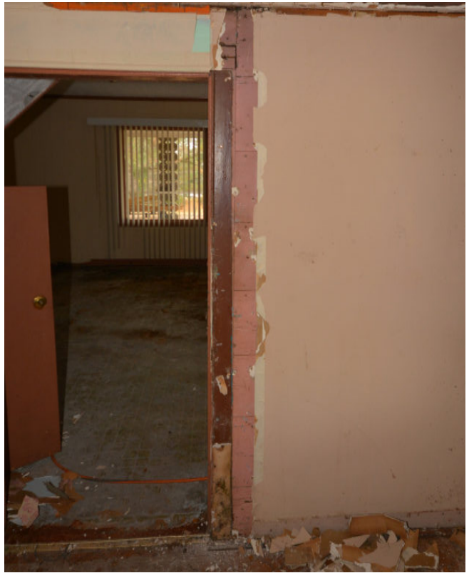
Figure 14: Corner bead door trim and tongue and groove wall boards exposed behind modern materials.
