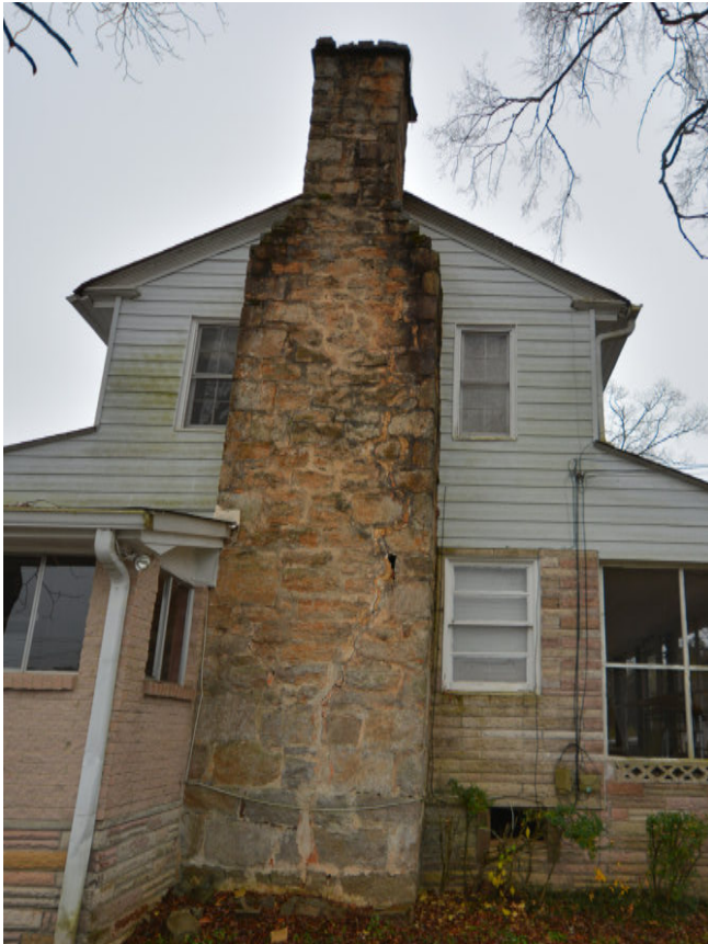
Figure 11: South chimney showing repaired crack.
