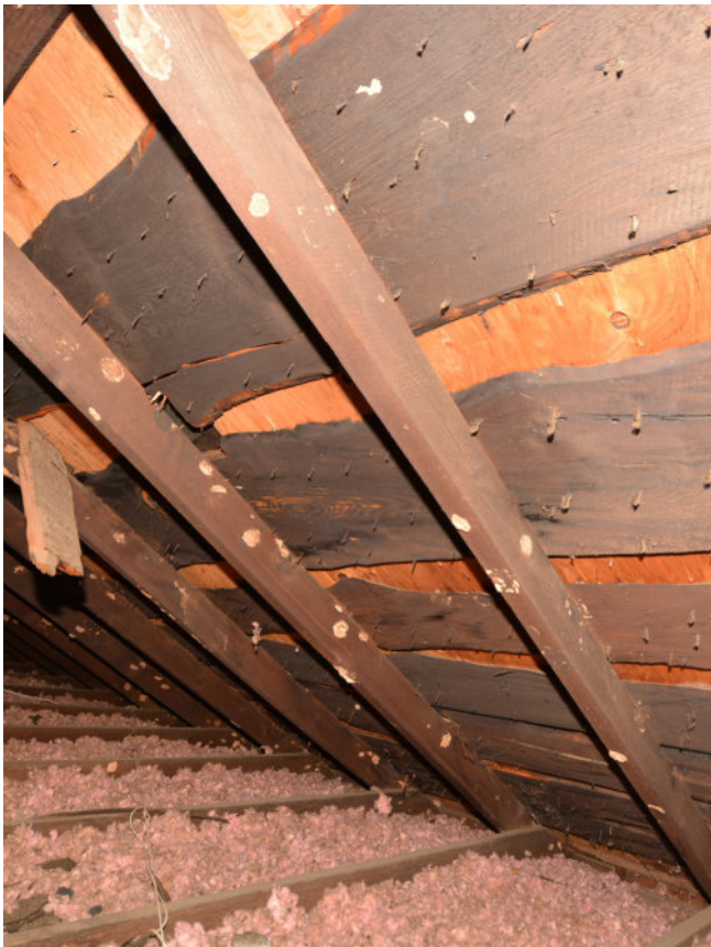
Figure 7: Typical roof framing and live-edge board decking.
