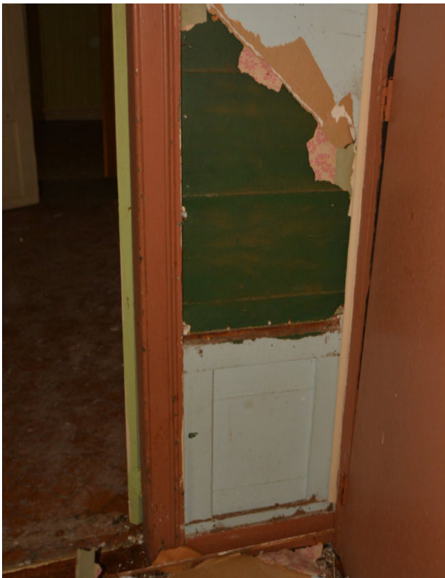
Figure 15: Tongue and groove wall boards above judge's paneling wainscot with original door trim to the left.
