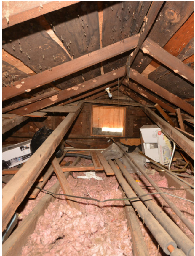
Figure 8: Gabled framing above sloped framing in the attic.
