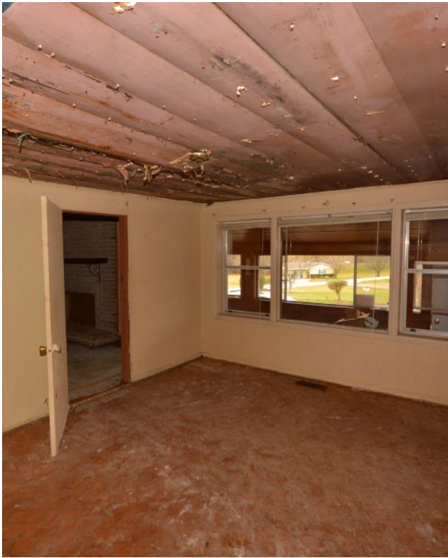
Figure 17: Exposed tongue and groove board ceiling.
