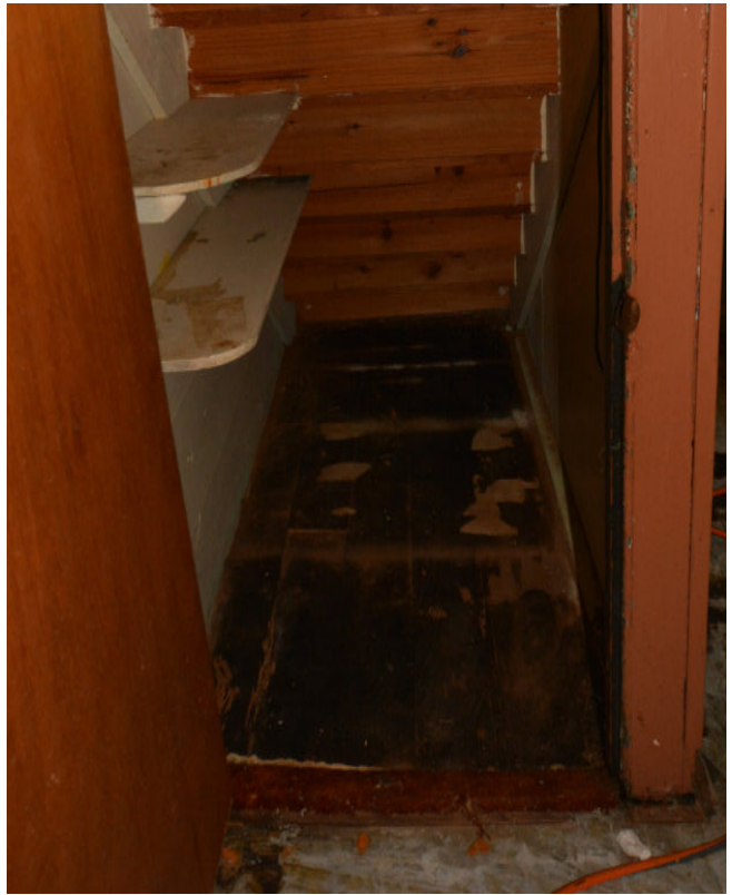
Figure 18: Exposed original flooring in original under-stair closet.
