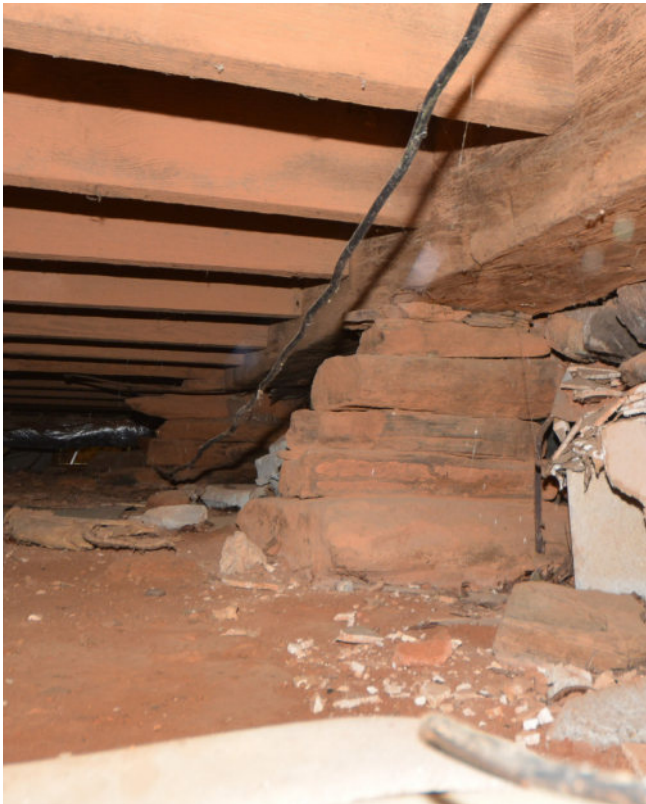
Figure 5: Stone foundation pile supporting large sill beam.
