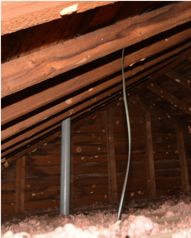
Figure 9: One of several locations where wood clapboards are visible.
