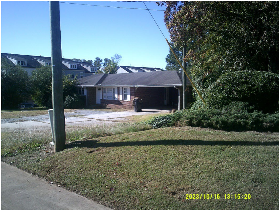
View of Existing Detached Single-Family Residence
