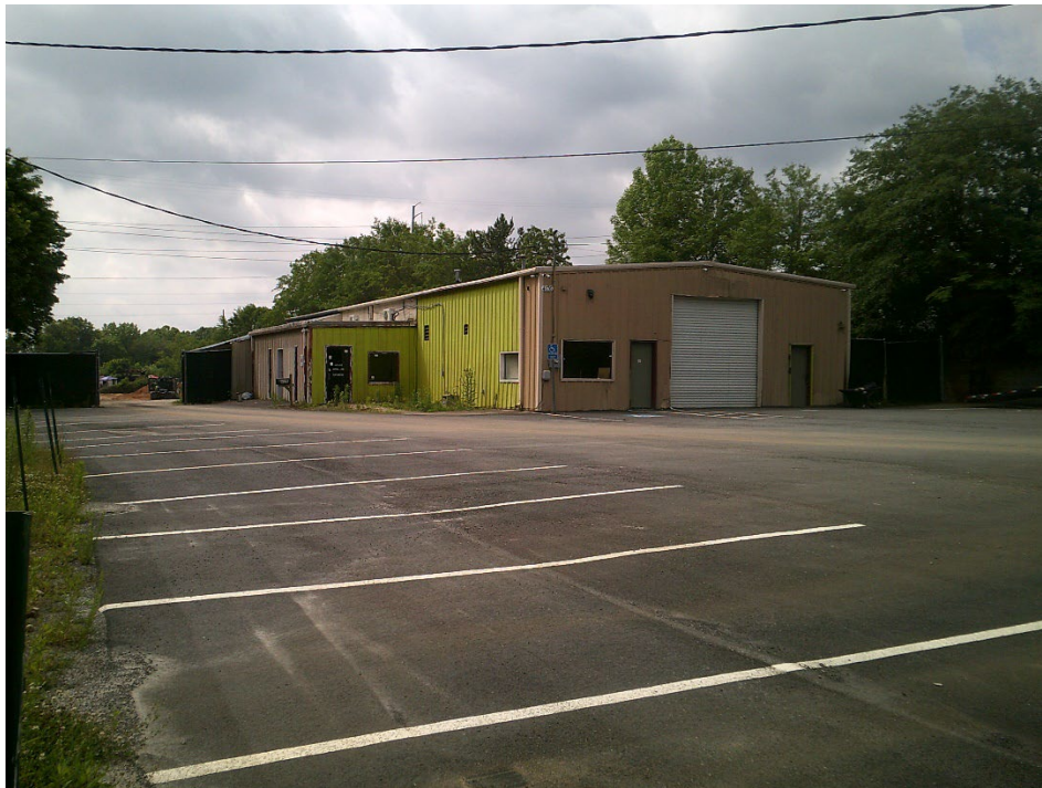
View of Existing Building from Parking Lot
