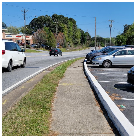
Existing sidewalk along Singleton Road
