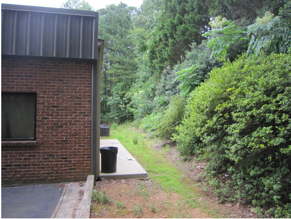
View of the rear of the building
