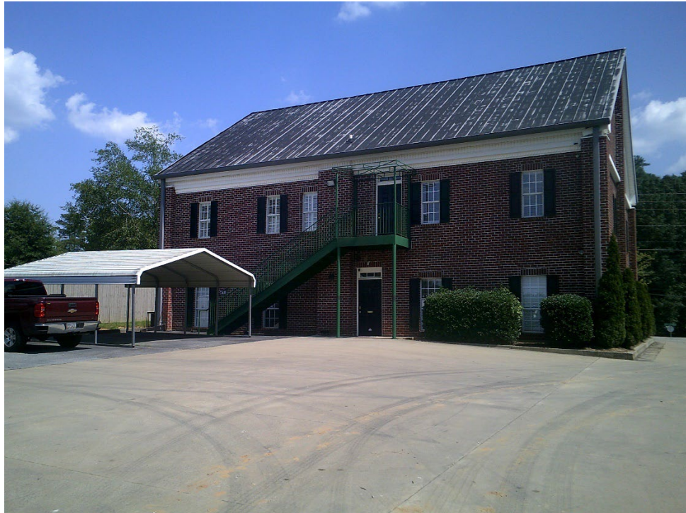
Rear View of Existing Office Building
