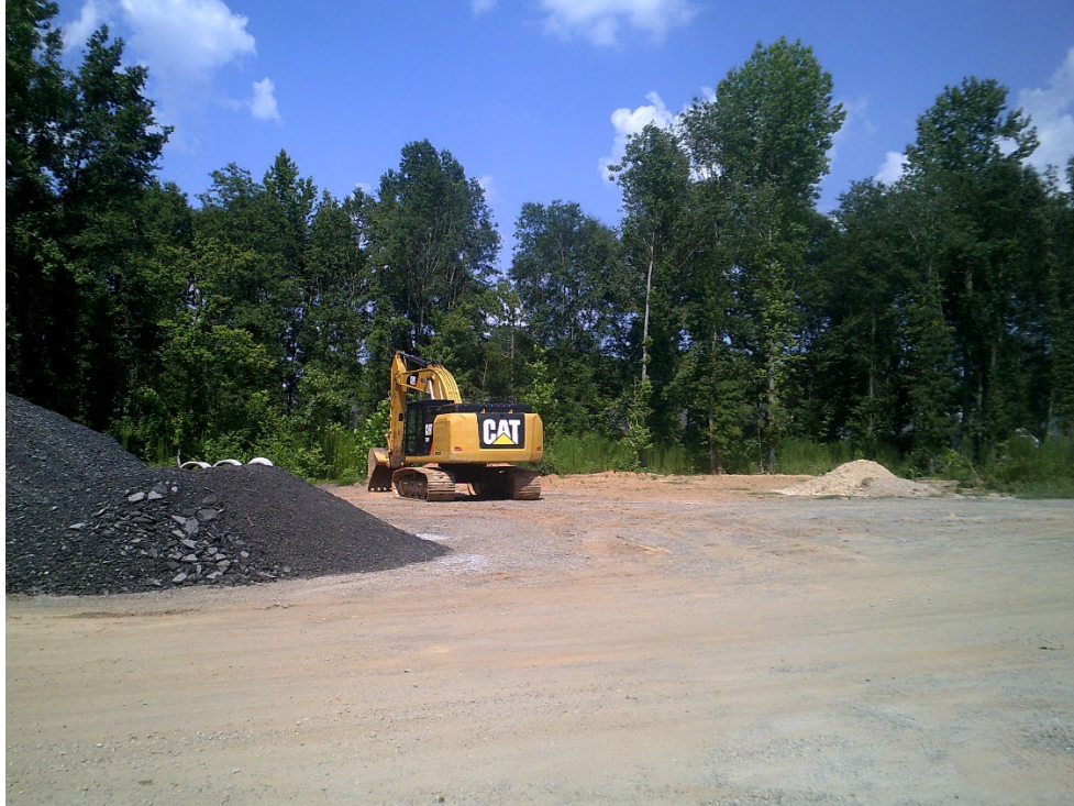
View of Machinery and Outdoor Storage Materials on Site
