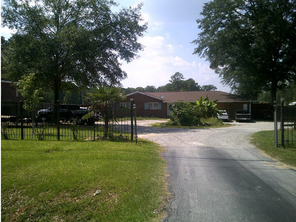
View of the Residential Structure Proposed to be Demolished
