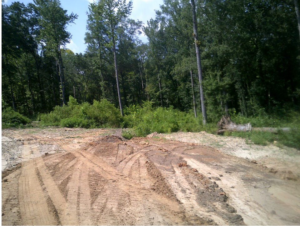
View of the Rear of the Site Towards Northwestern Boundary
