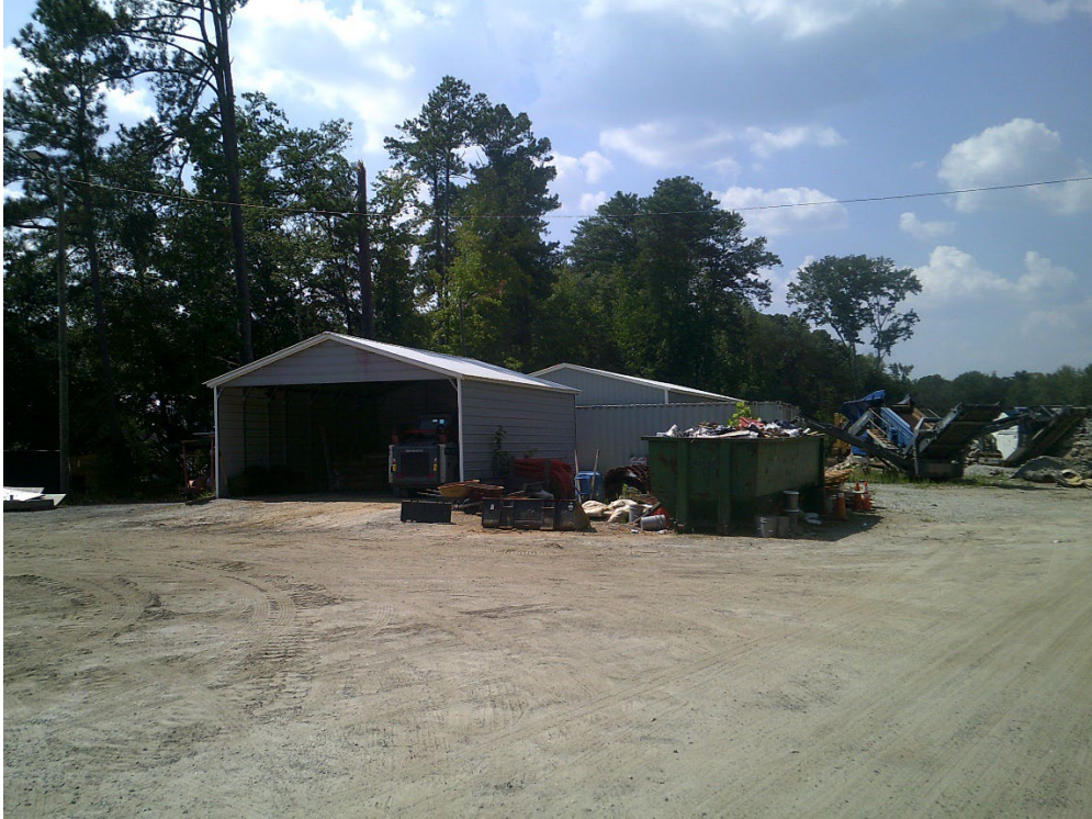
View of Accessory Structures and Outdoor Storage Materials
