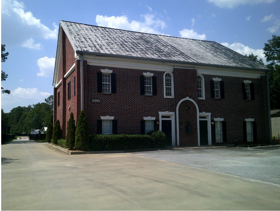
Front View of Existing Office Building
