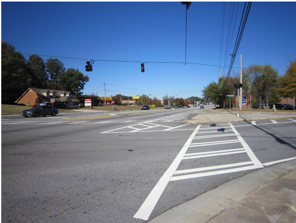
View of Centerville Highway and Zoar Church Road intersection facing north
