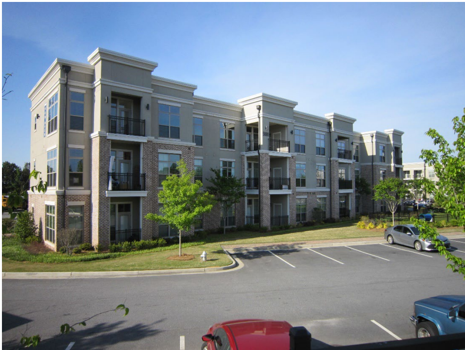
View of existing apartments immediately to the east.
