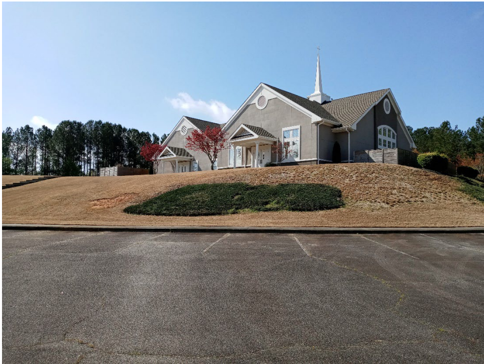
View of existing structures and parking
