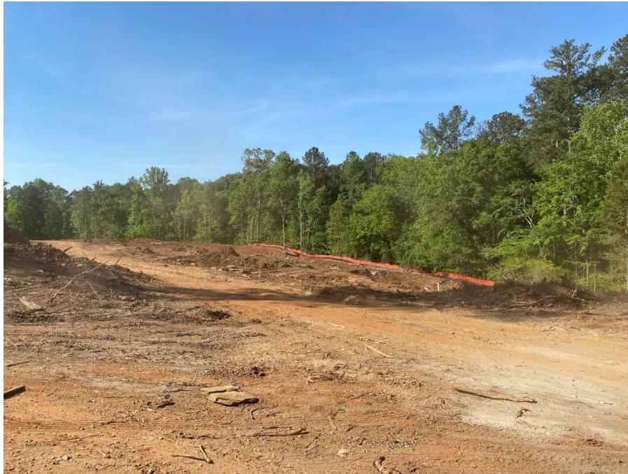
Main Drive into Subject Property from Winder Highway
