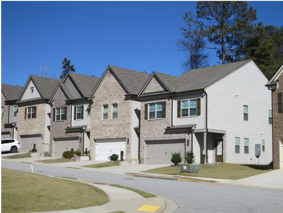
View of Norwich Place townhouses across Highpoint Road
