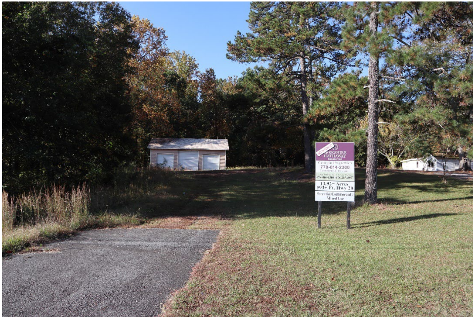
View of existing garage on subject property
