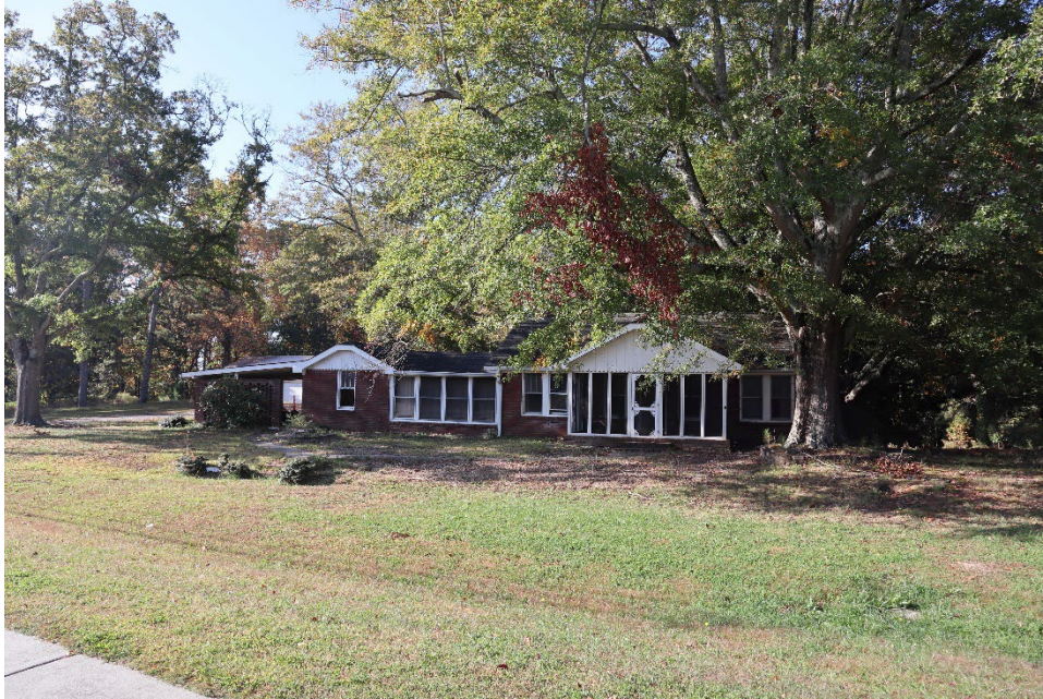
View of existing house on subject property
