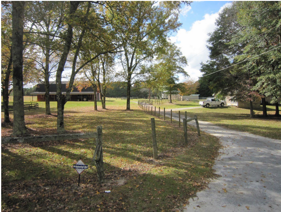
View of encroaching driveway into subject property and location of the proposed retaining wall
