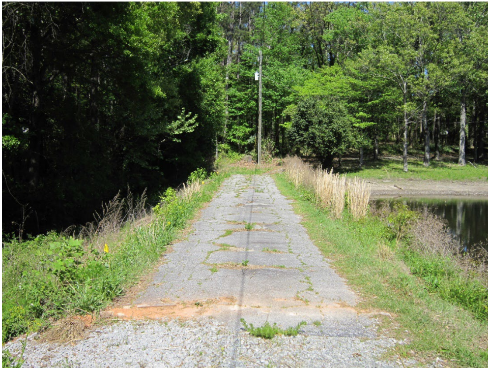
View of existing driveway beside the pond.
