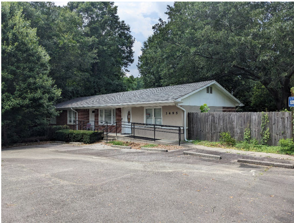
Existing Parking on Site
